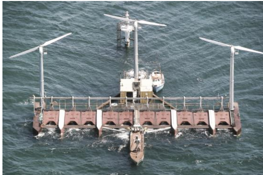
FLOATING POWER PLANT
